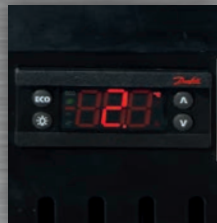
Danfoss controller with built in voltage protection
